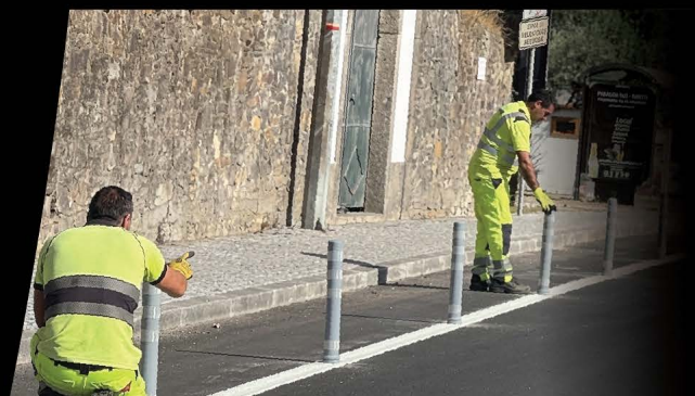
INSTALLATION OVER AN EXISTING MARKED CROSSING — NO LANE RECONSTRUCTION
