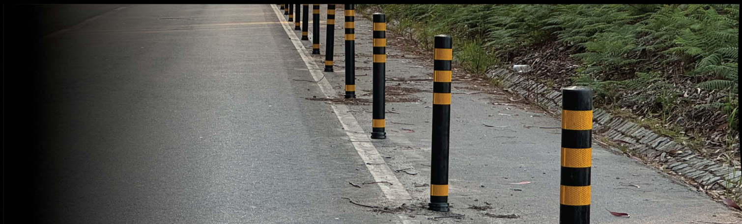
VERGE AND SHOULDER DELINEATION ON A RURAL ROUTE — 800 MM UNITS, BLACK BODY, FOUR YELLOW RA2 BANDS
