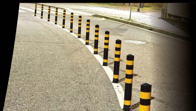
DUSK ON AN URBAN DISTRIBUTOR — FOUR RA2 BANDS KEEP THE LINE READABLE IN LOW LIGHT
