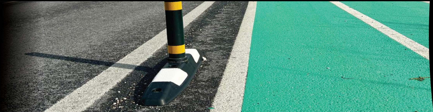
A continuous rubber kerb element with a rounded profile and four mechanical fixings, designed to carry a flexible bollard and separate a lane properly.
