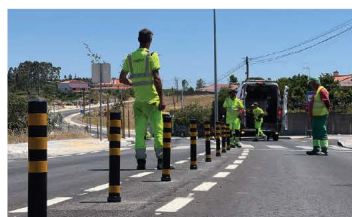
MEDIAN DELINEATION THROUGH A HIGH-SPEED CURVE — 800 MM UNITS AT CLOSE CENTRES HOLD THE LINE WHERE A RIGID BARRIER WOULD NOT FIT
