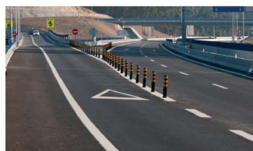
MEDIAN DELINEATION THROUGH A HIGH-SPEED CURVE — 800 MM UNITS AT CLOSE CENTRES HOLD THE LINE WHERE A RIGID BARRIER WOULD NOT FIT
