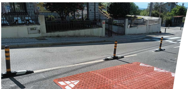
Bidirectional protected cycleway on an urban arterial - A Continuous, unambiguous edge at vehicle mirror height.
